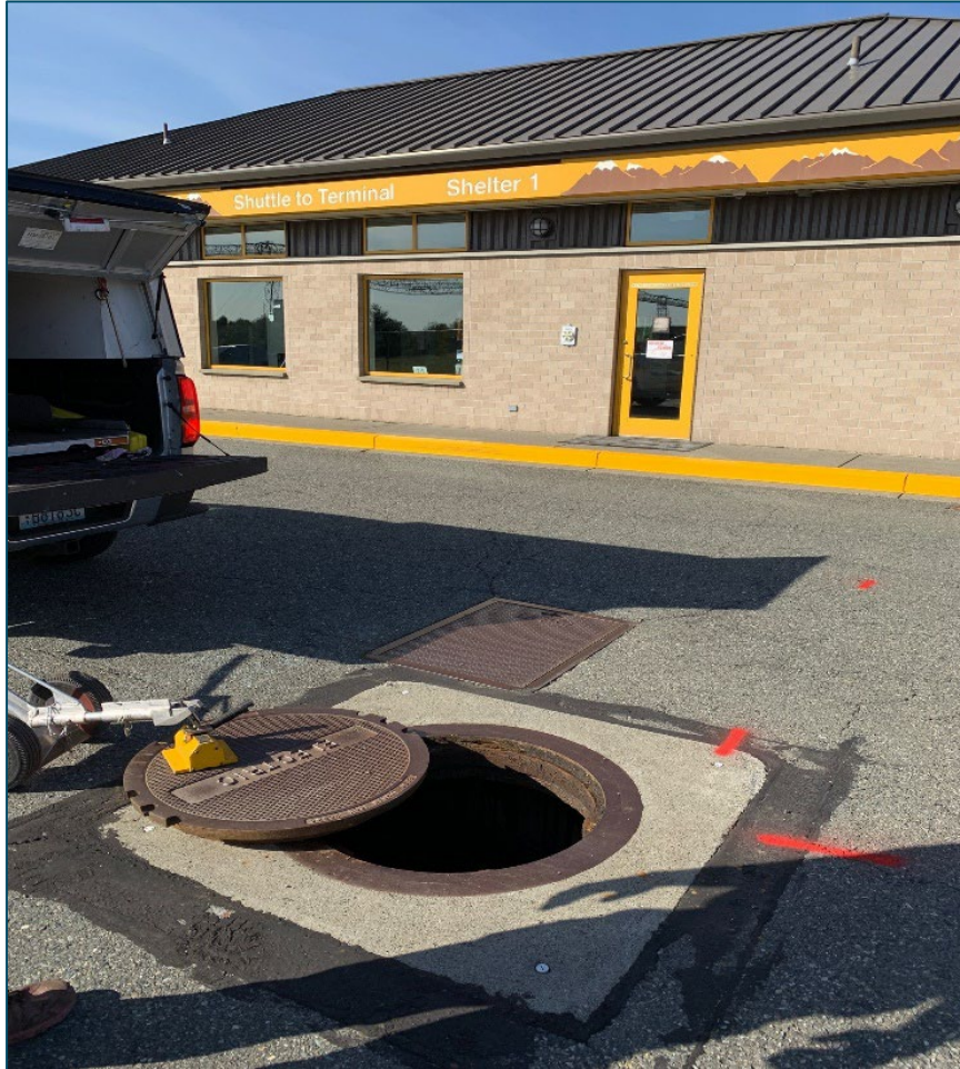
Electrical Vault at Shelter 1
