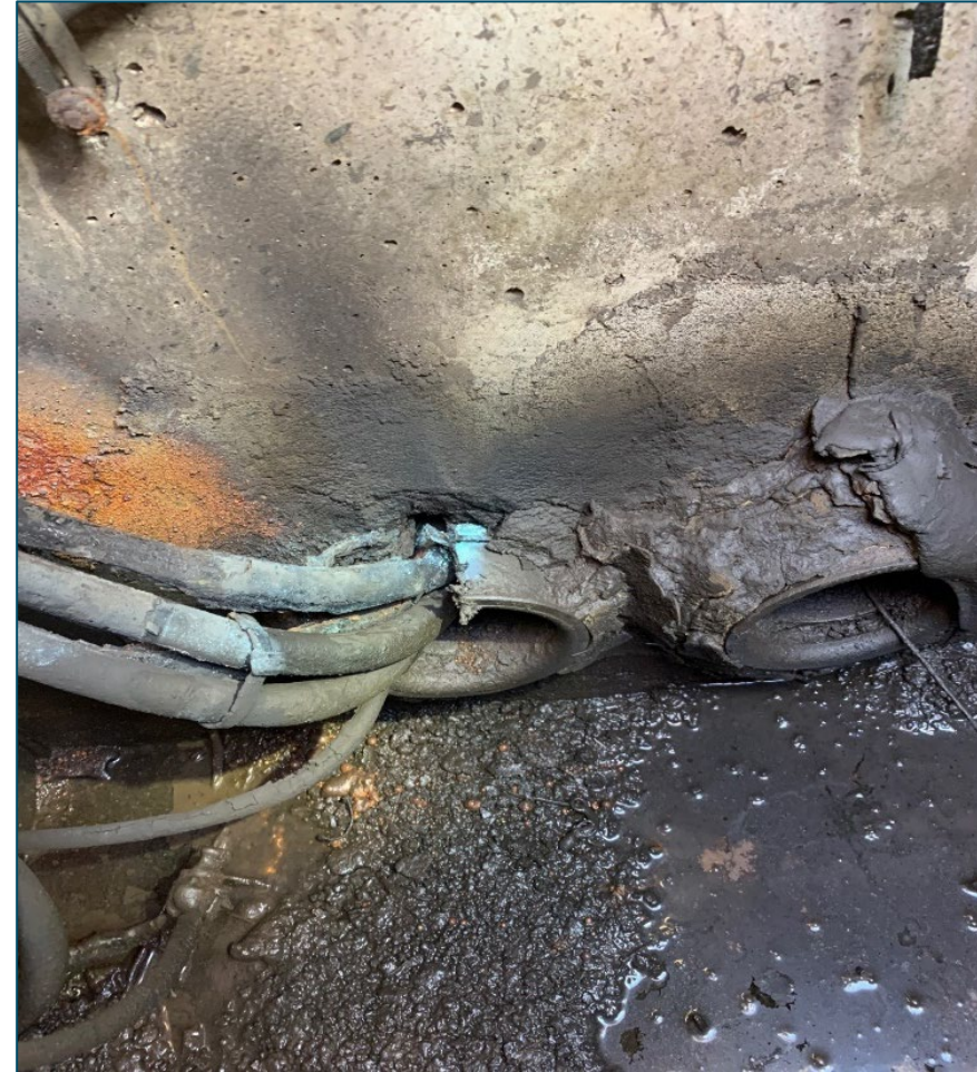
Failed Electrical Feeders to Shelter 1
